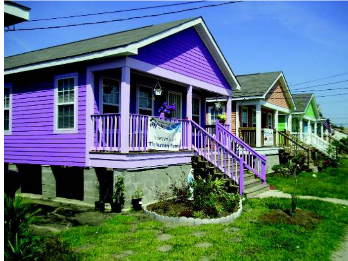
Figure 1 Houses with pier foundations recently constructed by Habitat for Humanity in New Orleans, Louisiana.
