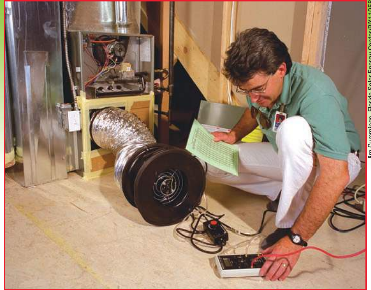
In this photo, a Building America staff member performs a duct blaster test to measure the impact of duct leakage on whole-house performance.
