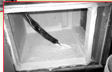
Repair of a platform return. Before (top): Note the cracks and gaps along the edges and joints. After (right): The same platform return after it has been sealed from the inside using mastic.
