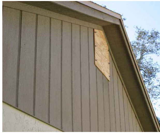
Figure 3.3. Outside shuttering of a gable end vent
