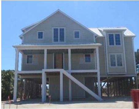
Figure 2.7. Post and beam/piling
