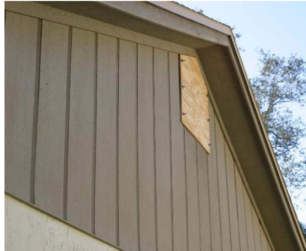
Figure 3.3. Outside shuttering of a gable end vent
