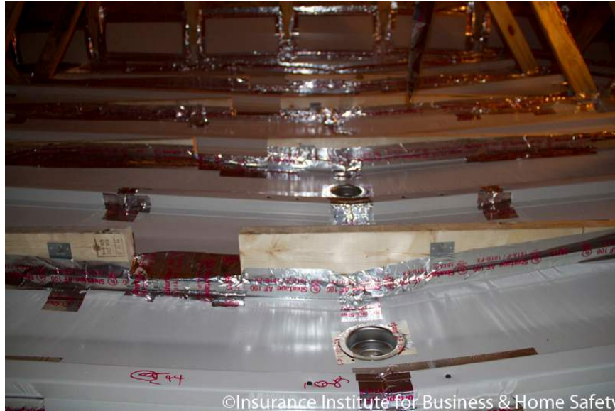
Figure 1. Photograph of water collection channels between ceiling trusses in duplex.
