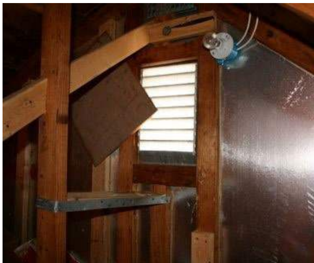
Figure 3.2. Example of a gable end vent with
