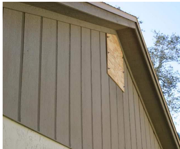
Figure 3.3. Outside shuttering of a gable end vent
